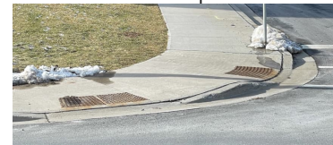
Example of Tactile plates at Pedestrian crossings for Accessibility (Dartmouth, NS)
