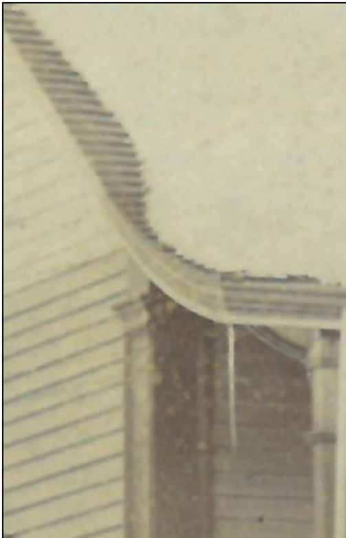
Return eaves prior to removal.
