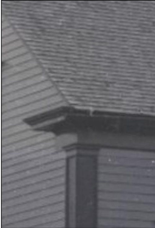
Return eaves prior to removal.
