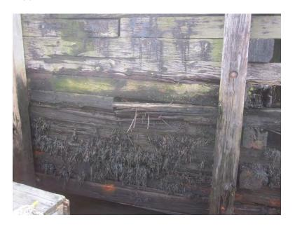
Photo 5: Severe deterioration of timber in tidal zone.
