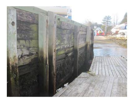
Photo 1: Displacement of Timber Crib Face
