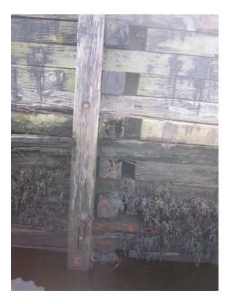
Photo 3: Ends of Cross Ties Shoreward of Area of Maximum Displacement
