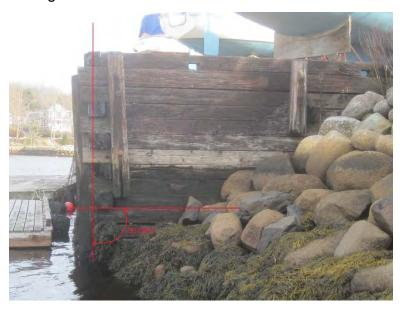
Photo 4: End of Cribwork showing Outward Displacement
