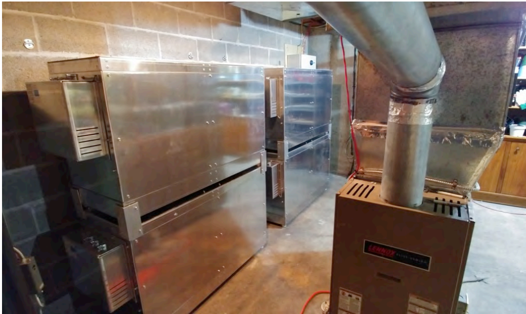
Neothermal ETS 2019 Prototype Integrated with Oil Forced-Air Furnace in Halifax, NS, CAN
